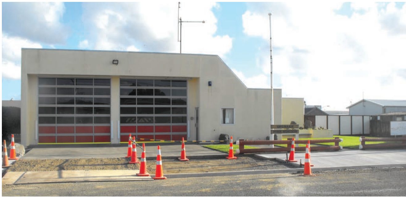
The new footpath in front of the fire station is still being developed.
